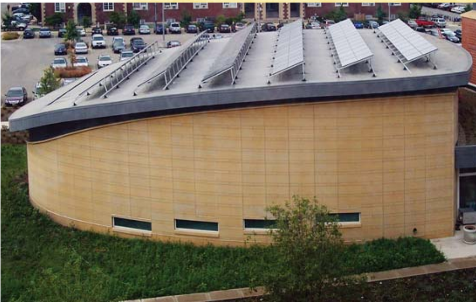
Photo: Business Instructional Facility, Urbana, Illinois - Winner of the 39 th Annual Engineering Excellence Eminent Conceptor Award (2010). Designed for the University of Illinois at Urbana-Champaign by KJWW Engineering Consultants
