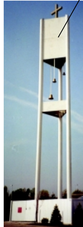
Church bell tower with antenna located behind tower panels
