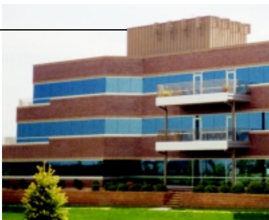
New building screen wall with antenna painted to match
