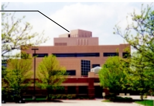
Antenna attached to existing building; painted to match
