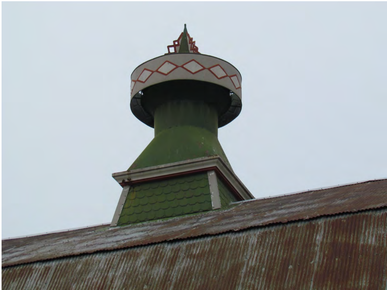
Figure 5. Modern or antique replacement roof ventilator on hog house (site 82-05979) on David C. and Melissa Hopson Evans Farm (site 82-05875), facing northwest. As shown in Figure 15, no roof ventilators were located on this building about 1960.
