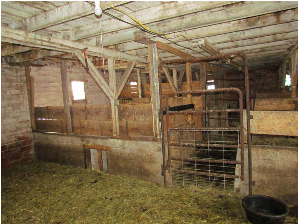
Figure 8. Interior of hog house (site 82-05979) on David C. and Melissa Hopson Evans Farm (site 82-05875), facing southwest. Low concrete walls with hog doors shown on both sides of the metal gate, with wood planking above.
