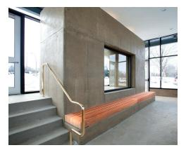
include the use of recycled steel and LED lighting fixtures throughout. Riders within the shelter can sit against the thermal mass and enjoy the warmth or coolness of the mass while an electronic sign displays arrival times of incoming buses.
